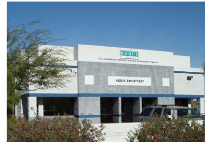
Hoque & Associates, Inc. facility at 4325 S. 34 th Street in Phoenix, Arizona
